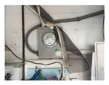
**Electrical Distribution Panels.** The building has an electrical distribution panel located in the pool manager's office. The panel separates the buildings' electrical power feed into separate circuits while providing protective circuit breakers for each circuit. The panel dates to the original construction of the building and has a rated service life of 50 years or more.
