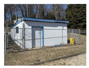
**Windows and Doors.** The Association is responsible for all of the facility's windows and exterior doors, which appear to be generally in fair condition. We noted corrosion on the main pool pump house door and frame. The pool manager's office door has deteriorated lower rails. The storage building's window and door appear to be in good condition.
