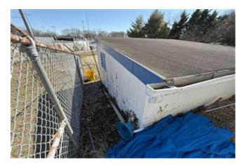
**Siding and Trim.** The buildings have wood soffits and trim, which appear to be in poor condition with damage and weathering. The wading pool pump house siding and trim appear to be in good condition.
